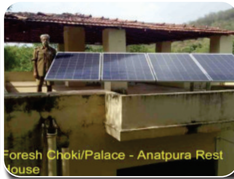
5HP SPV Water Pumping Systems, 1kWp SPV Power Plants for Lighting purposes at Forest Chowkies at Ranthambore Tiger Reserve
