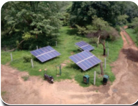
5HP SPV Water Pumping Systems, 1kWp SPV Power Plants for Lighting purposes at Forest Chowkies at Ranthambore Tiger Reserve
